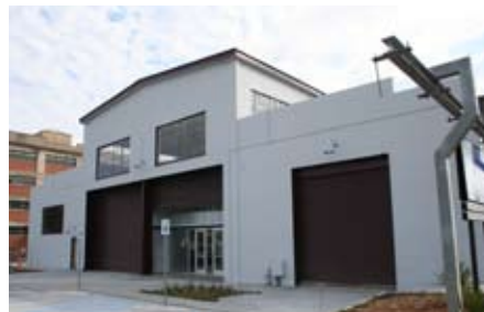
This warehouse in South Carolina is used by a trade school and a variety of local artists.
