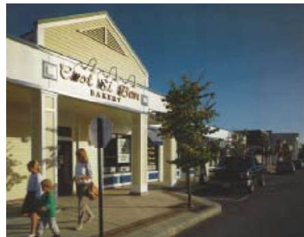
Shops must provide a variety of parking options and remain accessible by foot.
